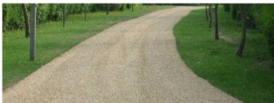
Tar Spray and Chip Surface Dressing
